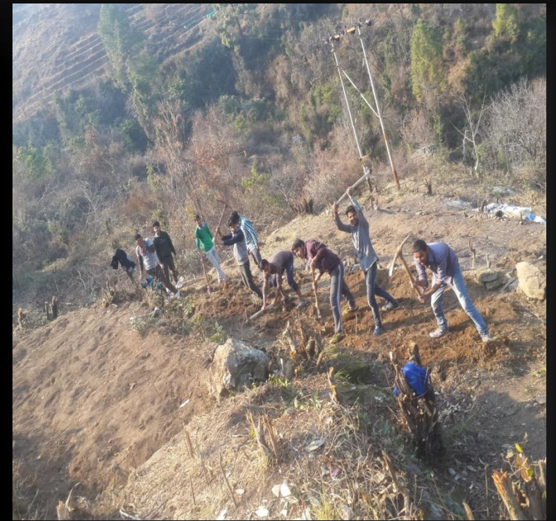
Leveling of field.
