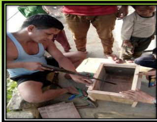
Construction of side walls by the help of needles & hammer.
