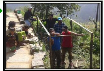
Construction of roof with the help of wild bamboo sticks
