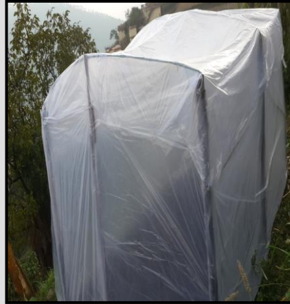
Construction of polyhouse of dimension 3.5x2.5 m 2
