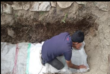
4. Covering the wall & sides
