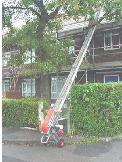
Plate : 19.2 Petrol engine operated Hoist
